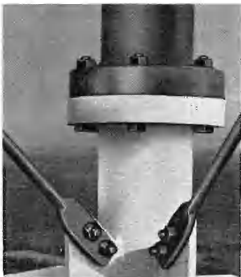
FIG. 10. Tower leg flanges are precision welded for snug fit and ease of erection.
