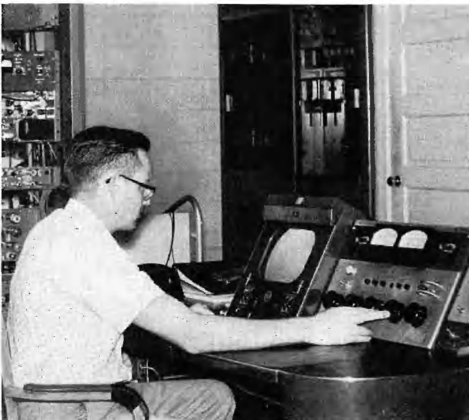
FIG. 12. WTVM transmitter plant. In foreground is the TTC-5 Control Console. At far background are the rectifier and control cabinets for the TT-25CH aural power amplifier.
