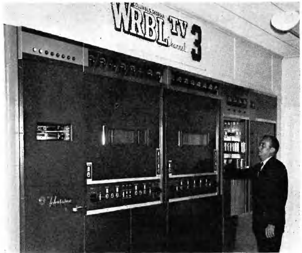
FIG. 8. WRBL-TV employs 25-kw Type TT-25CL TV transmitter.
