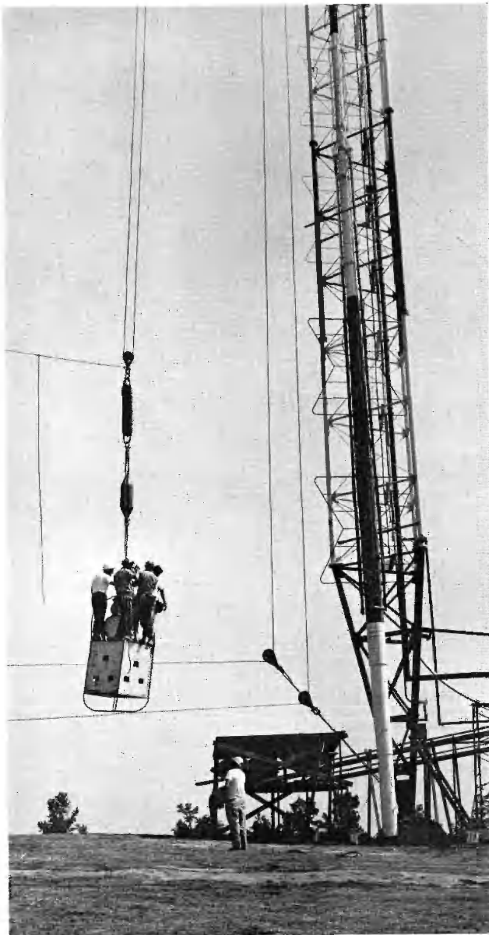
FIG. 5. Riggers used this temporary elevator car (tool basket) to ascend and descend the tower during the extension of tower height.
